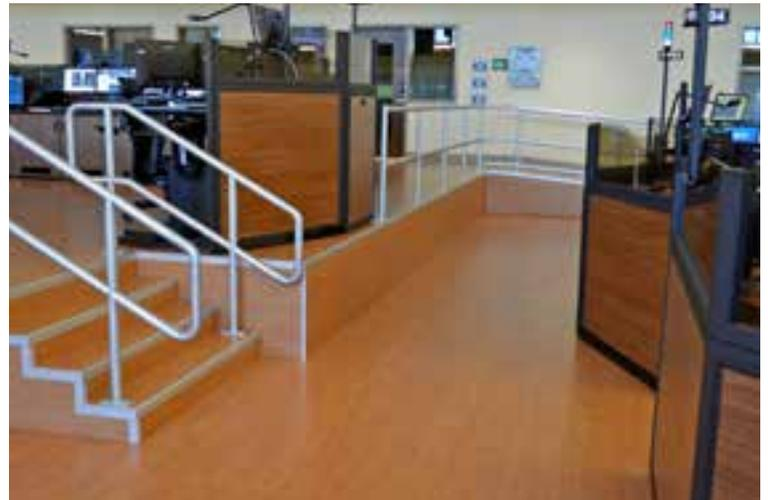
The flexible and adaptable Iso Floor construction allows de- signing for loads of up to 800 lbf/sf (40 kN/m<sup>2</sup>.) Distances between support members (Lx, Ly, Lz) are the factors guiding the static design load.
