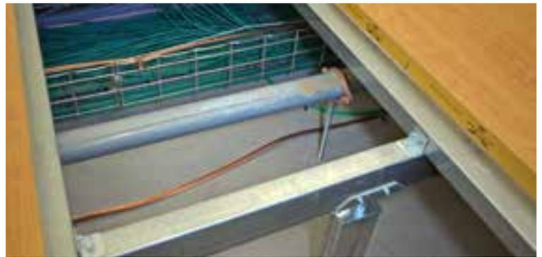
Bergvik's Iso Floor for the 911 Dispatch Center was built in two levels, with a 18 & 42 inch (450 & 1065 mm) finished floor height to provide a higher Supervisor platform area in the center of the dispatch center.
