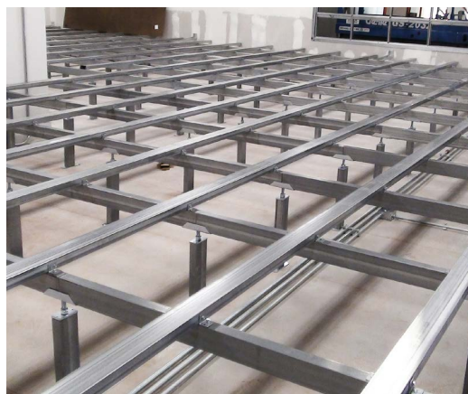
Transformer Room at Karolinska Hospital with reinforced Iso Floor Substructure supporting 16 Transformers with a total weight of 120 ton.
