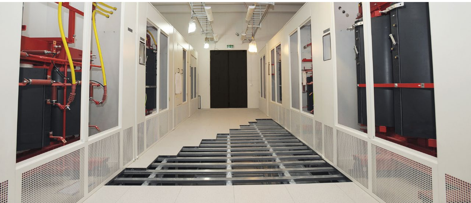
Transformer Room at Karolinska Hospital with reinforced Iso Floor Substructure supporting 16 Transformers with a total weight of 265,000 lbs (120 tonnes).
