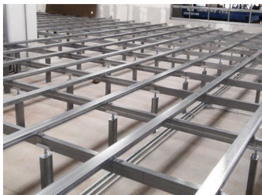
Transformer Room at Karolinska Hospital with reinforced Iso Floor Substructure supporting 16 Transformers with a total weight of 265,000 lbs (120 tonnes).
