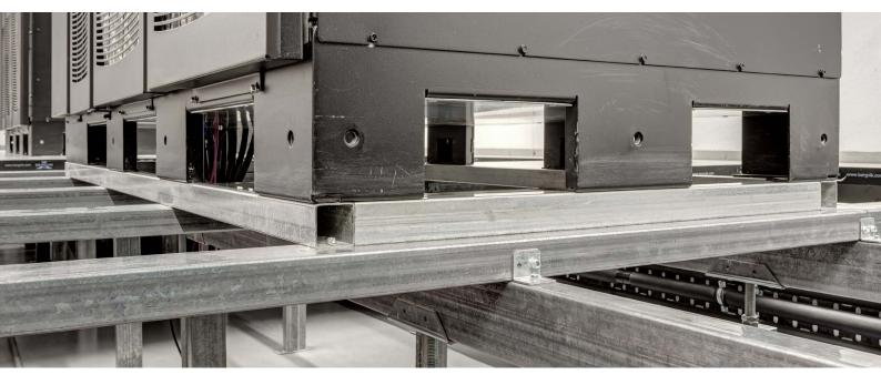
Simply build any electrical equipment support frame by bolting 40x40 tube steel directly on top of the standard Iso Floor substructure. Years later when you upgrade e.g. PDU's, CRAH's or Battery Racks and they have a different footprint, you just adapt the 40x40 tube frame and you are done at a minimal cost. Major time and cost savings!
