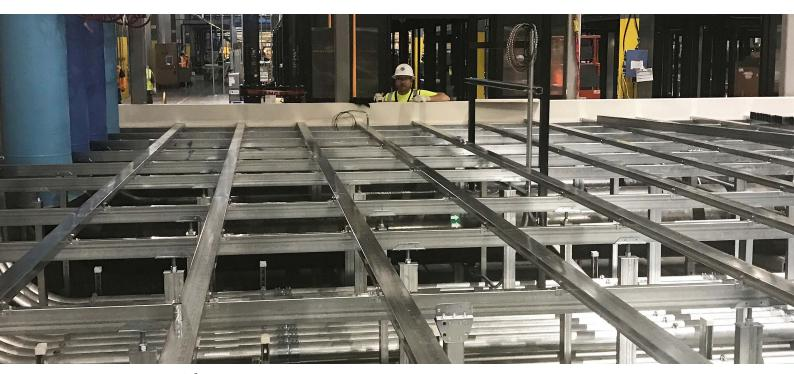
Iso Floor supporting 36.5 kN/m<sup>2</sup> of electrical equipment for a major technology company in Arizona.
