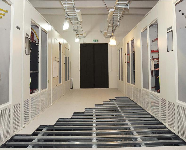
Transformer Room at Karolinska Hospital with reinforced Iso Floor Substructure supporting 16 Transformers with a total weight of 120 ton.
